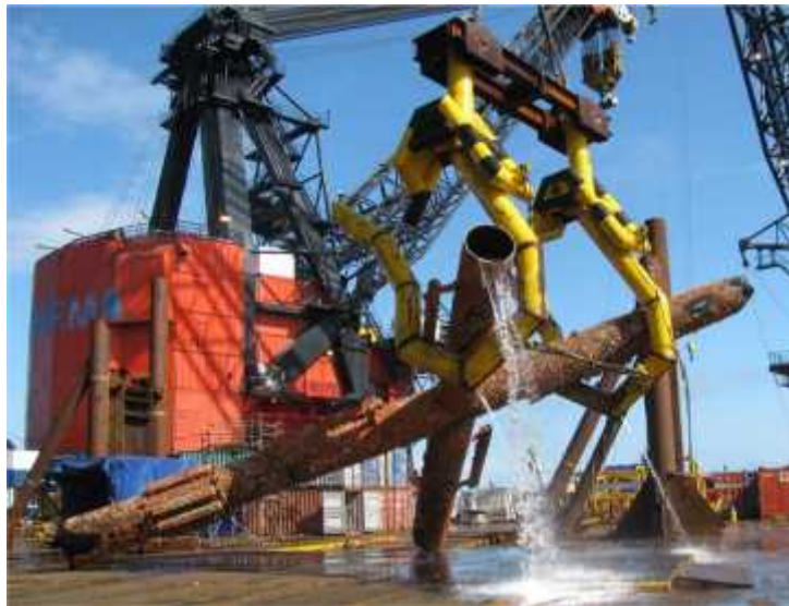
Figure 16: Section of Jacket Lifted Using Clamps
