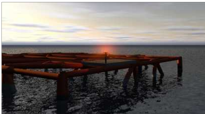
Figure 7: Jacket left in situ after removing topsides
