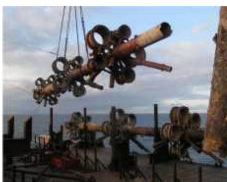
Figure 17: Backloading Jacket Sections onto Barge
