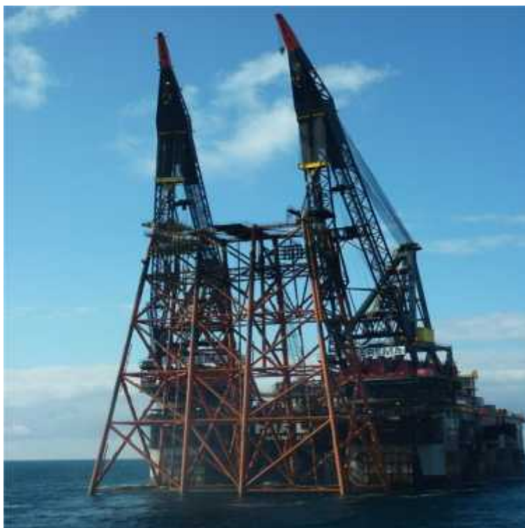
Figure 8: Jacket Removal using SSCV
