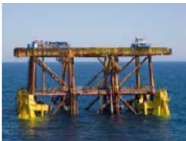
Figure 18: Refloating the DP2 Jacket using BTA's
