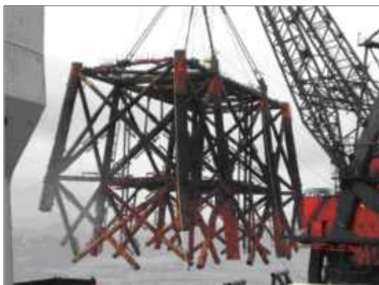
Figure 12: Removal of Jacket Section
