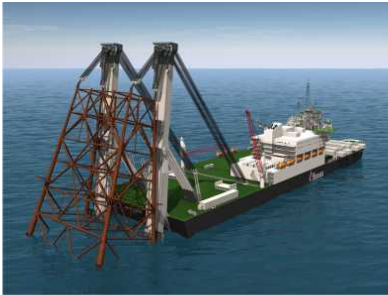
Figure 9: Jacket Removal using SLV
